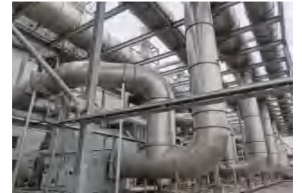
VOCs waste gas treatment facilities
